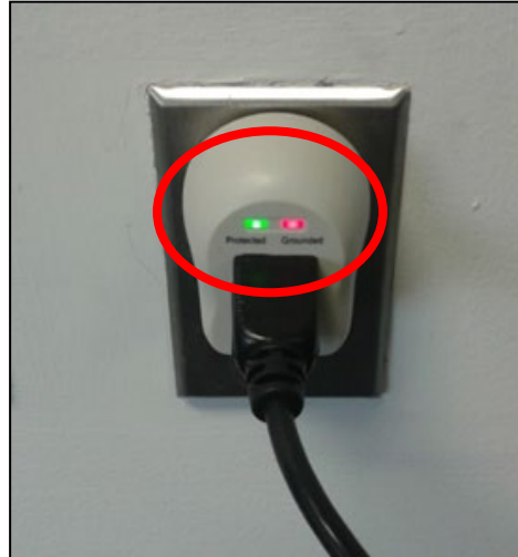
Figure 5 - Picture of Red and Green Lights on the Surge Protector
